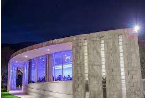
Three Rivers Memorial Building
